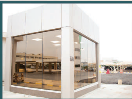
Establishing an external common room in King Fahad Medical City
