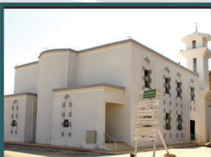
Building a Mosque in Al-Makhwah
