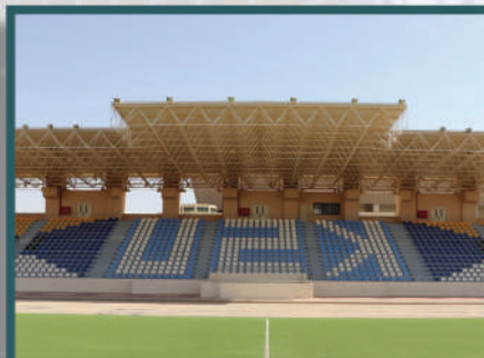
Rehabilitation of sports and ambulant area of King Saud University
